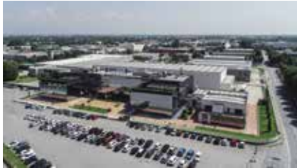
MP FILTRI Headquarters in Milan
